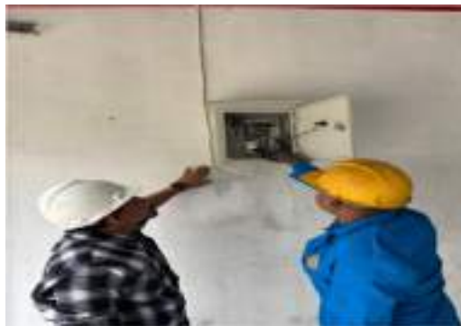
Gambar 5. Gambar Pengecekan Ulang Panel
